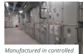
HTM 03-01 compliant AHU
