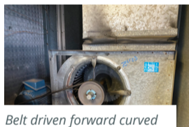
Belt driven forward curved fans
